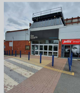
This one's Through a service yard!
