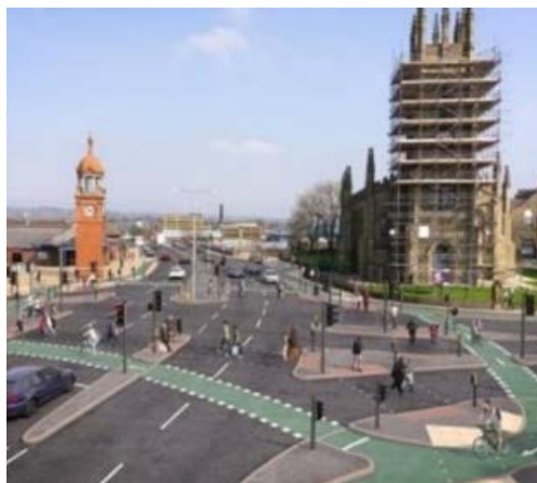
Bolton: Junction upgrades
